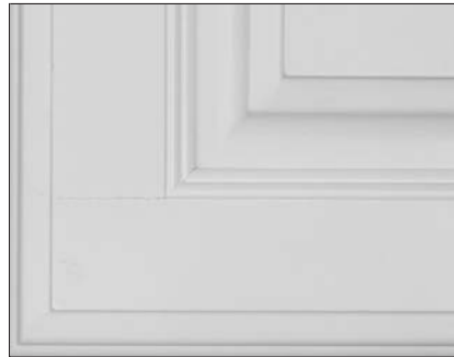
Example of door front joint separation
