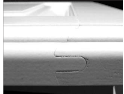
Example of door end joint separation
