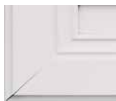
Separation of Door Corner
