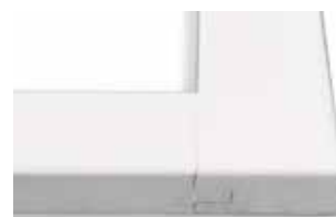
Separation of Door End
